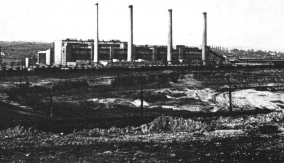
The Tisová power station, near Sokolov
